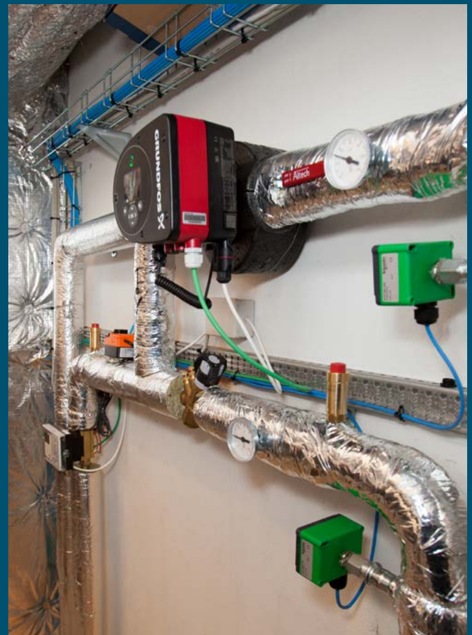
Strandby Skole, energirenovering.
